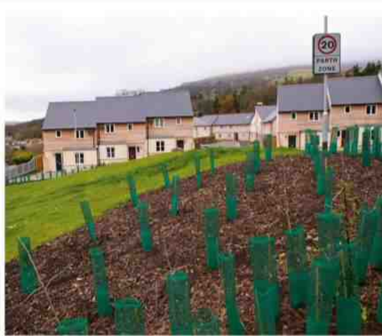
The building of new low-cost homes, such as these in Powys, Wales, is essential to boost rural economies, says CPRE
